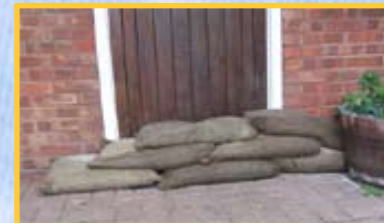
Floodbags used as a wall structure
